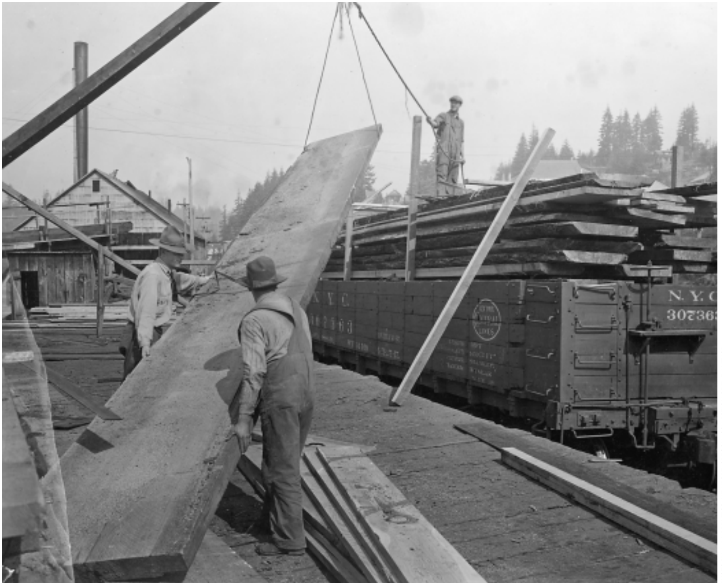
Loading spruce lumber onto a rail car at the Warren Spruce Company, Portland, Oregon. The wide boards were shipped to airplane manufacturers.
