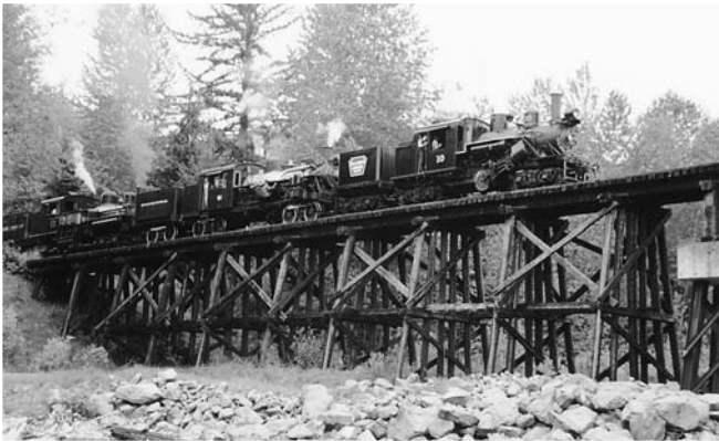
The 3-truck Climax #10 (left) crossing the Nisqually River trestle.
